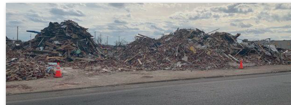
Downtown Mayfield KY Damage
